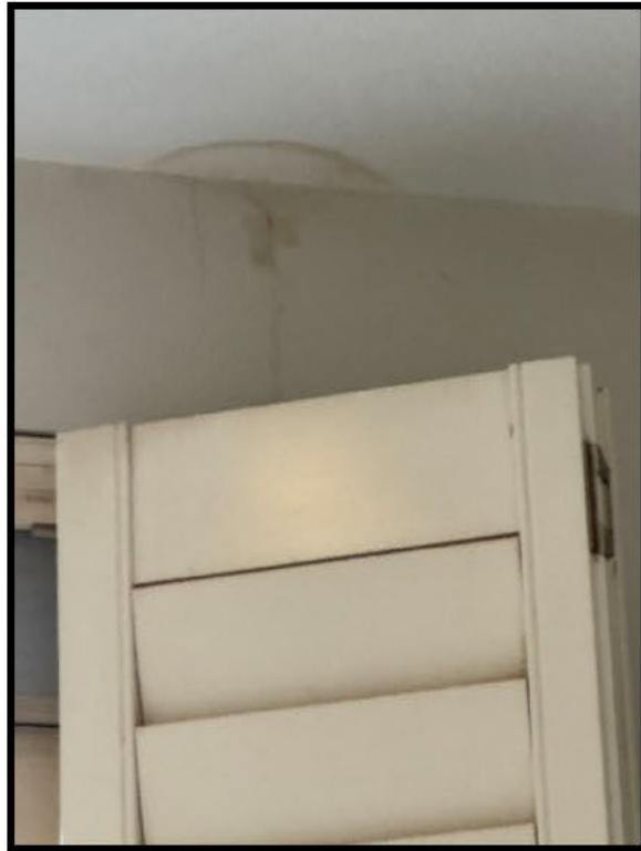
Damp stain to ensuite bathroom ceiling
