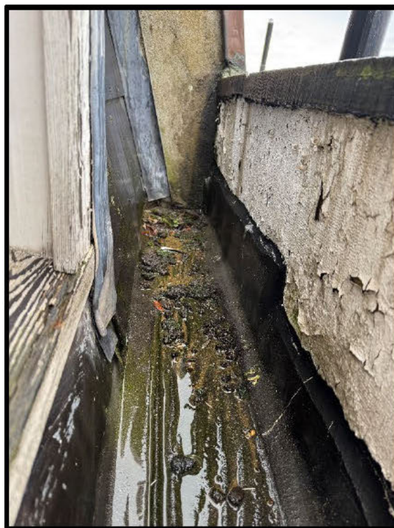
Part blocked parapet gutter – please note the condition of the gutter lining which is showing indications of deterioration and will form a repairing obligation in the short / medium term
