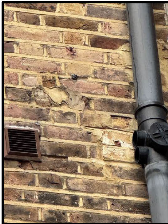
Damaged upper brickwork to the rear elevation
