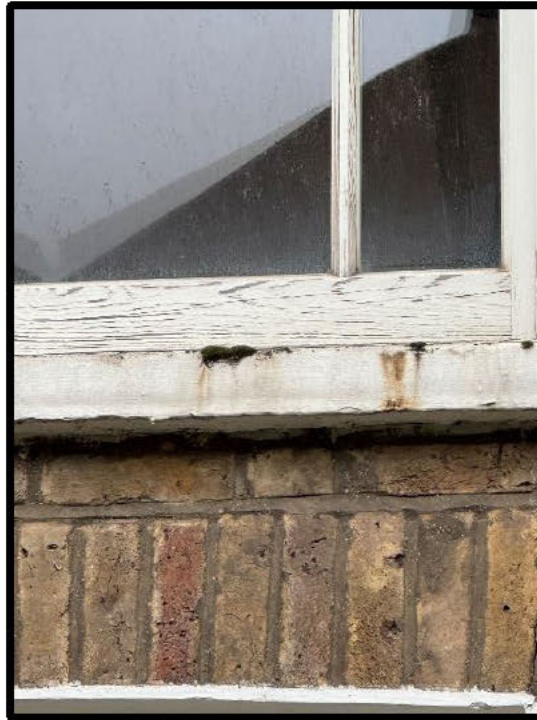
Poor decorations and damaged sill to the rear elevation
